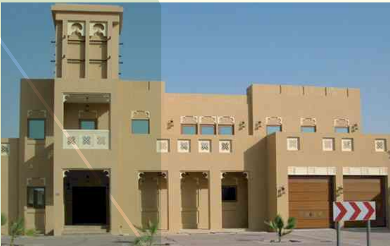
Jumeirah Park Villas, Dubai - U.A.E Partial Electrical Works
