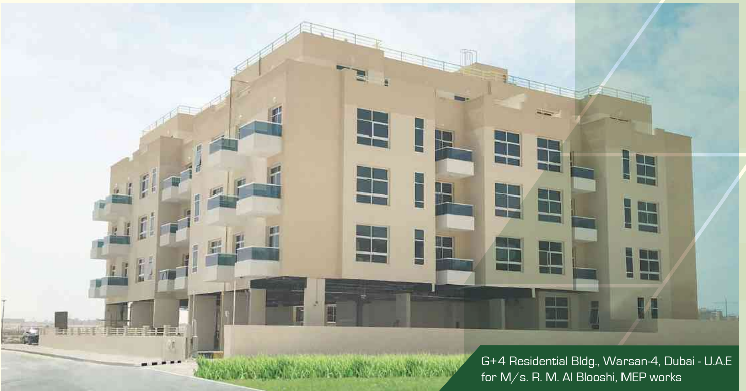
G+4 Labour Accommodation, DIP-2, Dubai - U.A.E for M/s. Royal Mega Interiors, MEP works
